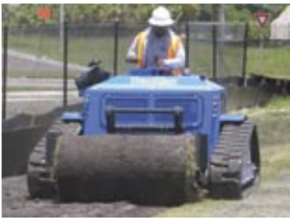
Sod installation is simple!
